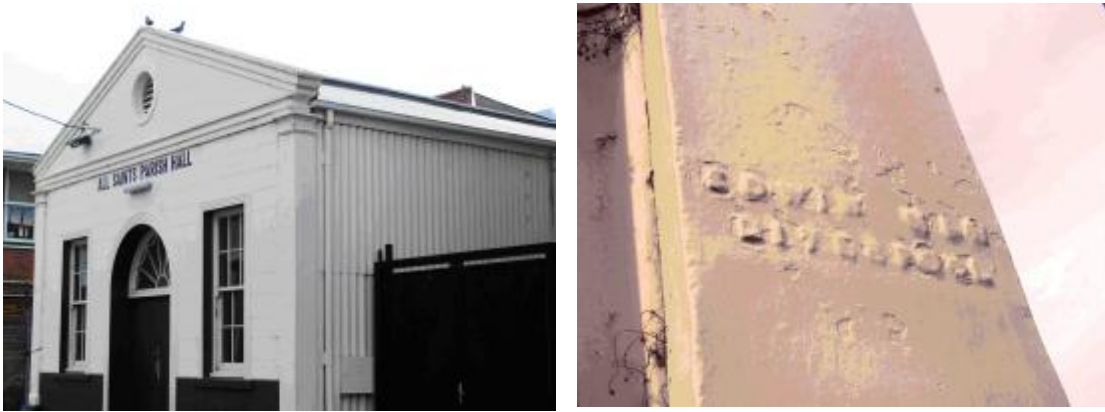
Building in King William Street, Fitzroy, believed to have been a store or warehouse of about 1853, later All Saints Parish Hall: view and detail, of the brand 'EDWIN MAW LIVERPOOL'. Miles Lewis
