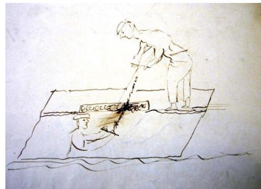
The garden layout (for the purpose of constructing a railed fence), and 'Used the cross cut saw and got a fine chopping log placed in the kitchen', Beale diary, 19 February 1840, 11 March 1840. The diagram shows pit sawing.
