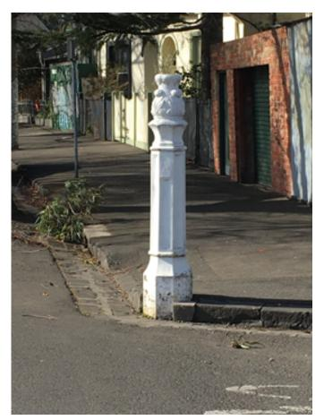
A typical gas light standard. The upper column has been removed and the remaining standard filled with concrete. Electric lights were mounted on replica gaslight standards around 1990 each with a single light source and mounted on a 4-6 sided glass lamp head.
