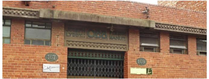
(This photograph, shows the decorative projecting cornice of pressed cement with a square crystalline pattern, repeated over the entrance (O.B.B. above the door stands for Oily, Black and Brilliant –the product manufactured in the factory)
