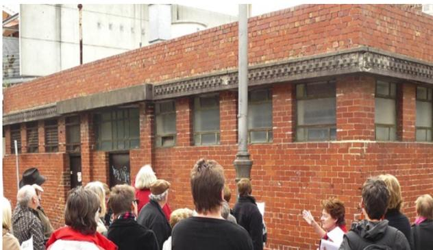
Tour guide, Willys Keeble pointing out the ribbon of windows punctuated by thick piers and a continuous decorative projecting cornice of pressed cement.
