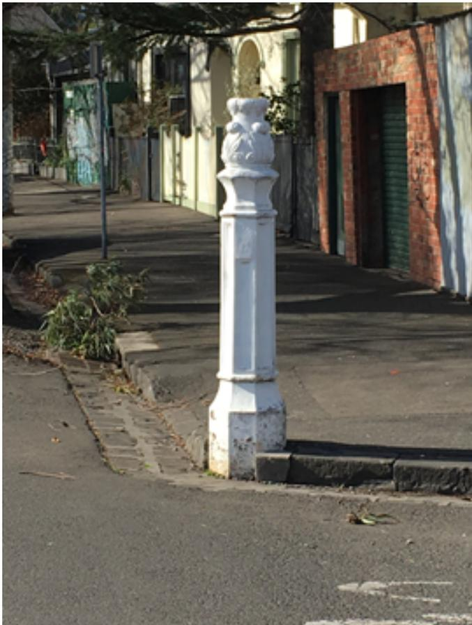
*A typical gas light standard. The upper column has been removed and the remaining standard filled with concrete. Electric lights were mounted on replica gaslight standards around 1990 each with a single light source and mounted on a 4-6 sided glass lamp head.*
