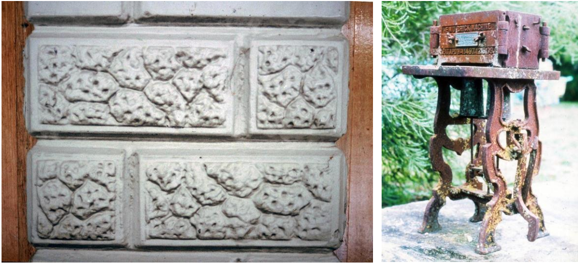
Midget Giant concrete blocks from Foster's Coffee Palace, Maffra, Victoria, 1908. 'Emu Brick Machine Pat Appd., No. 1149742509 [sic]', 'D. & W. Chandler Sole Agents Fitzroy' David Watson.
