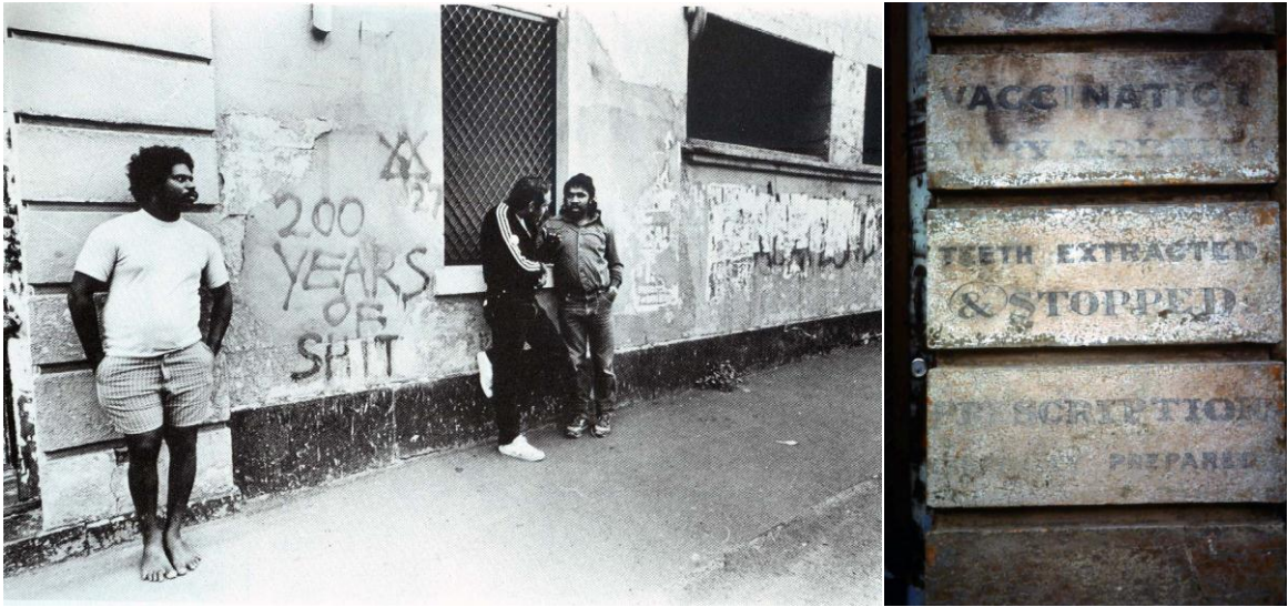
'200 years of shit', on the north side of Royal Terrace, 1988. Philip Castle photograph, Fitzroy Photographic Collection. Remains of original signwriting on the north wall of Dr Crook's surgery: Miles Lewis.
