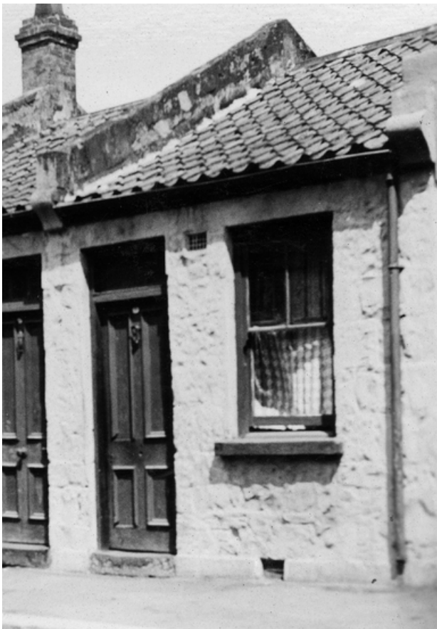
Jo studied Dr Sue Kee who lived at 2 Marion Street, Fitzroy and will talk about her research. This photo of terrace houses on Marion Street is from the State Library taken in 1935 before the houses were demolished (it may not be number 2).
