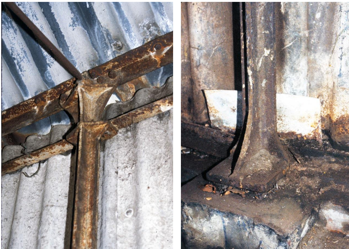
The Yarra Council building, head and foot of a stanchion: Miles Lewis.
